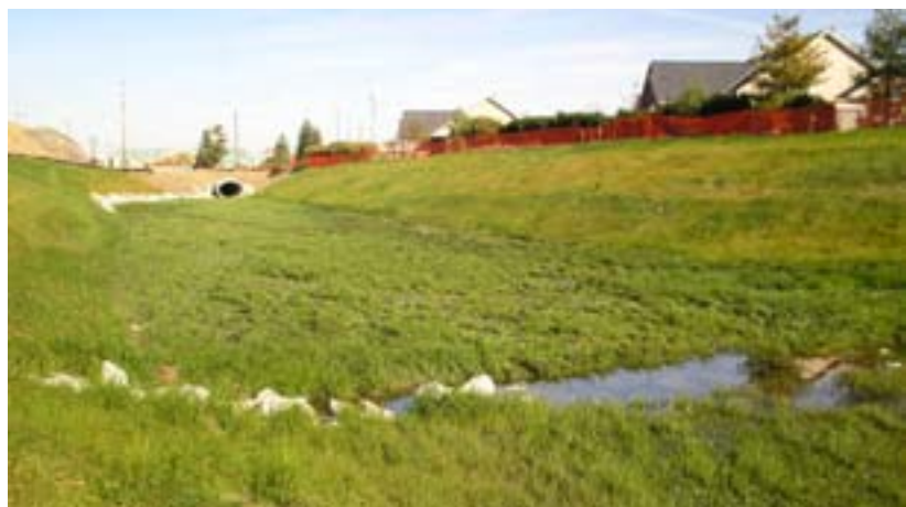
Application of over-wide channel technique. Source: EMH&T
