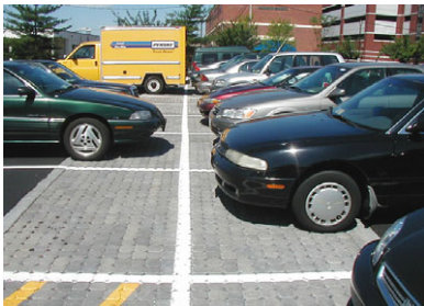
Example of Pervious Pavement Blocks, Washington, DC
