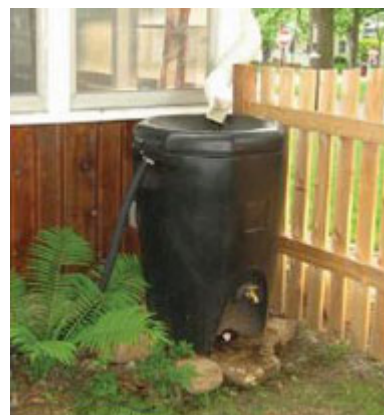
Example of Rain Water Harvesting Residential rain barrel — Stillwater, MN
