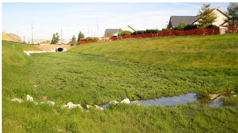
Application of over-wide channel technique.
